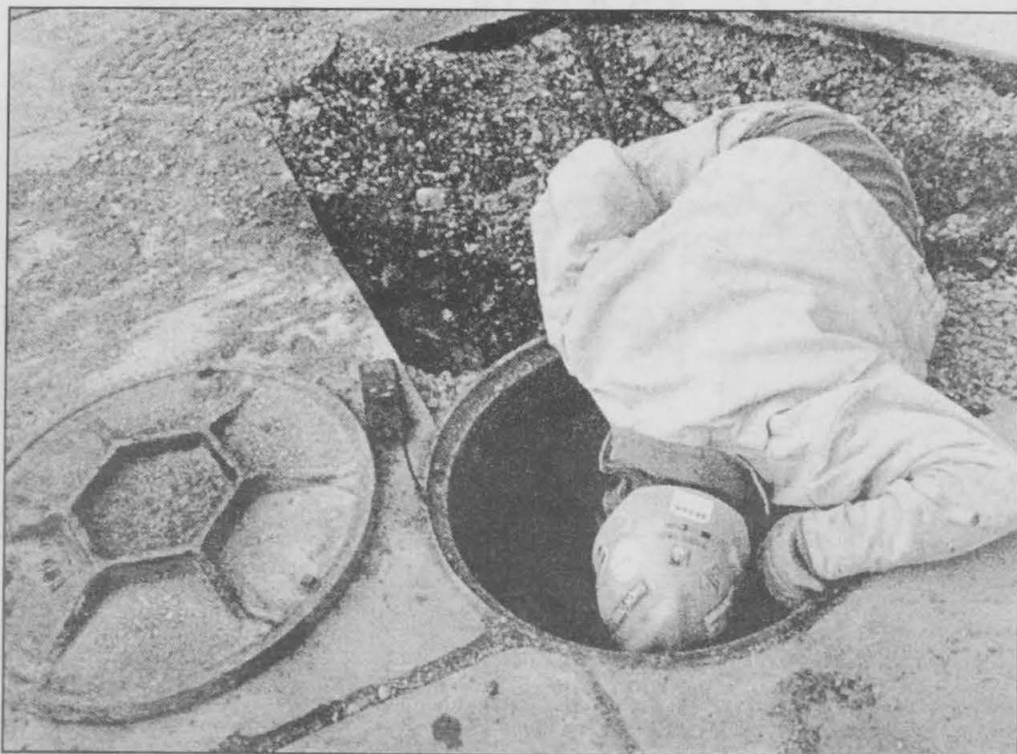
Threading a broad-band cable to a co-worker, Joe Harr puts the finishing touches on the steam tunnel near Howard Hall.
