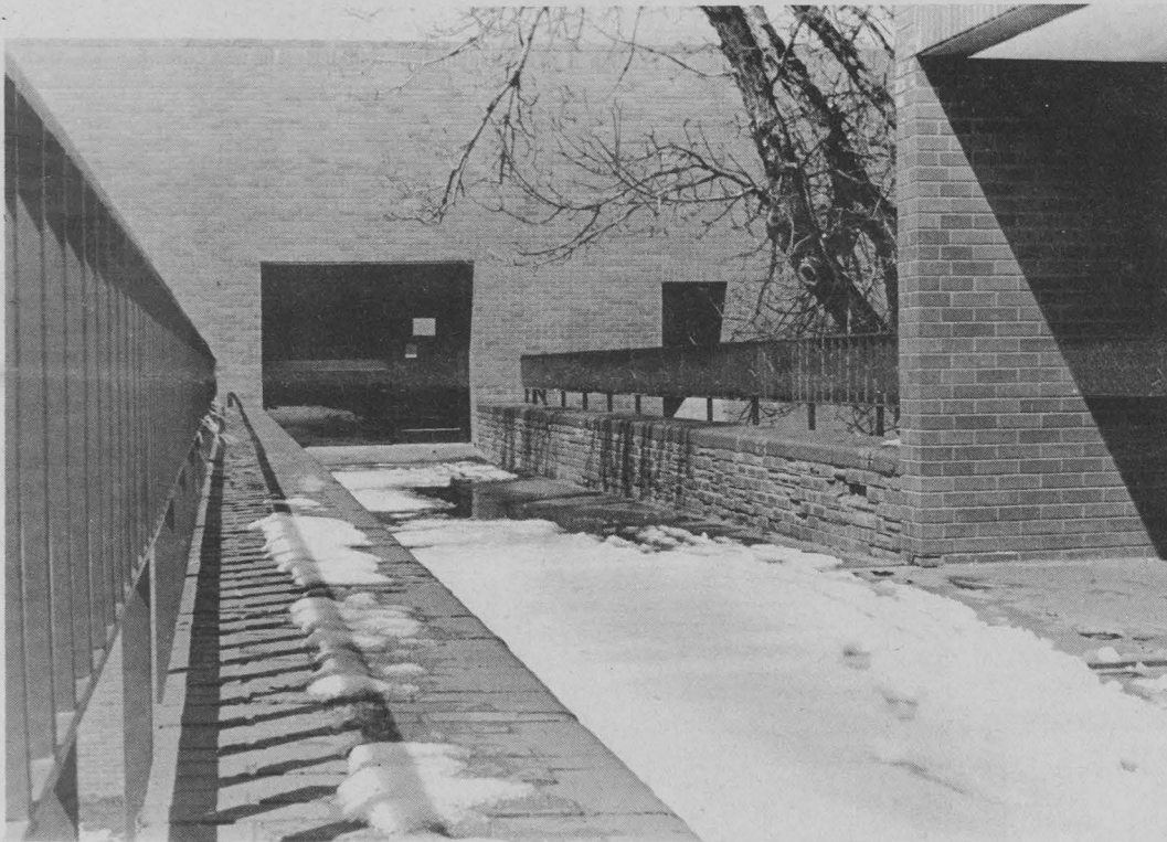
Improvement of walkways and handicapped access is a major part of MSU's Master Plan, which was adopted two years ago. (Staff photo by Dave Smith)
