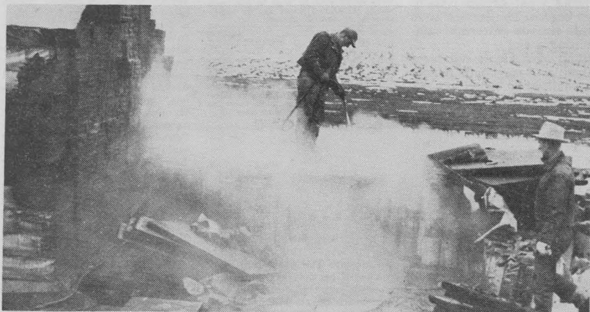
FALSE ALARM —What looked like a fire in MSC's new fieldhouse Tuesday morning turned out to be merely the accidental burning of some roofing
