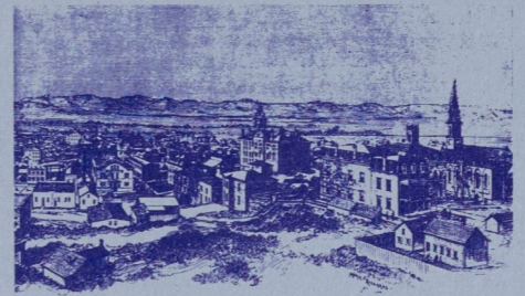
A GENERAL VIEW OF HELENA FROM FIRE TOWER HILL - 1887
