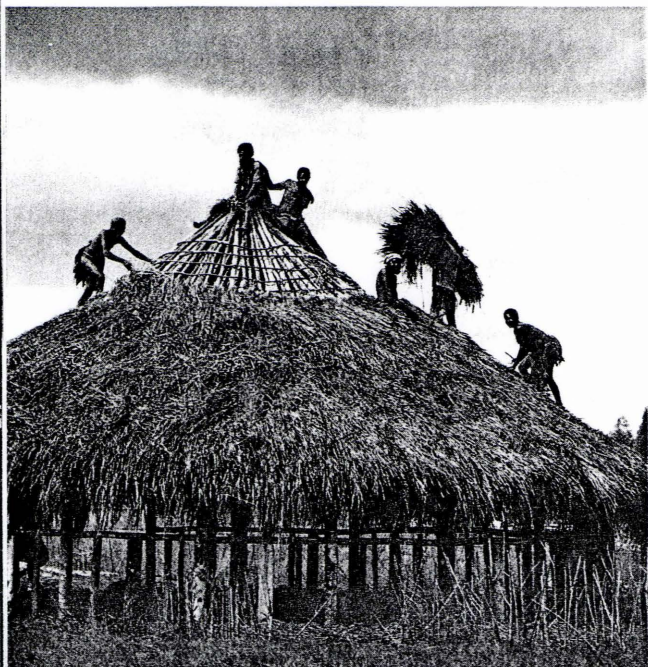
Villagers complete the thatched roof of a house built on piles in the interior of eastern New Guinea.
