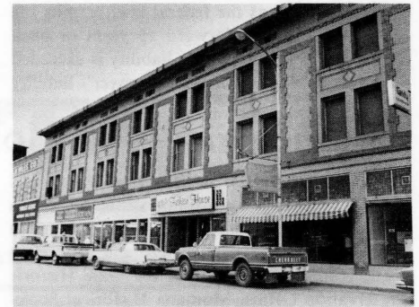
A. W. Miles Building
