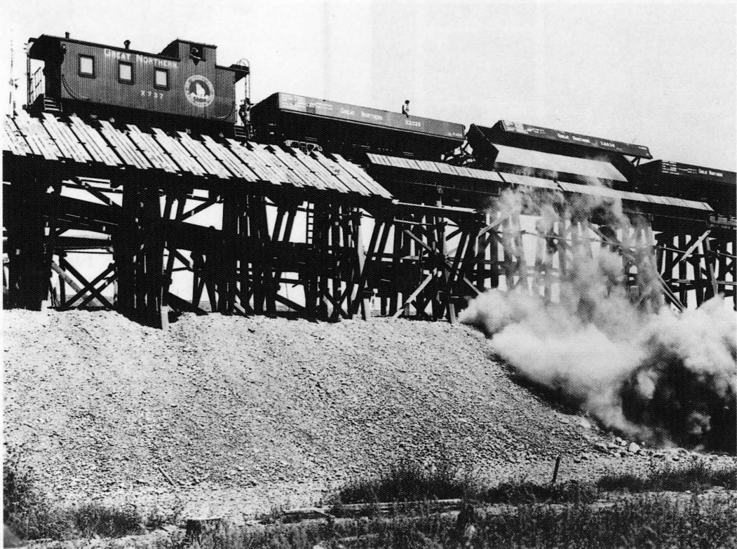
GRAVEL DUMPING INTO UPSTREAM TOE OF FORT PECK DAM, JULY 19, 1935.
