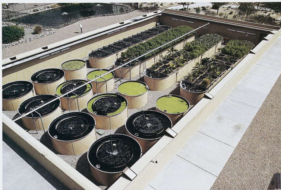
Effluent from Ethel M Chocolates in Henderson, Nevada, is treated here. Microbes in the foreground tanks begin the job; plants in the tanks at the rear finish it.
