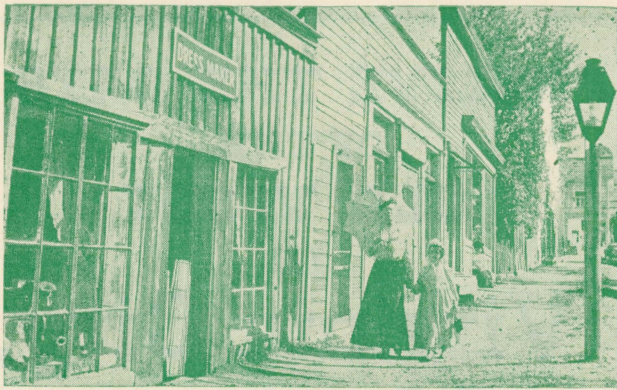
Board Walk, Virginia City, Montana
