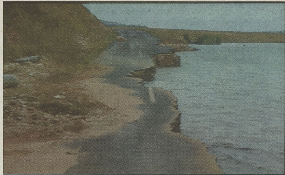
The 1959 earthquake caused parts of Hwy. 287 to fall into Hebgen Lake.
