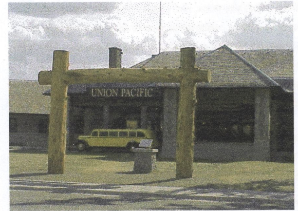
Yellowstone Historic Center in the Historic Union Pacific Depot
