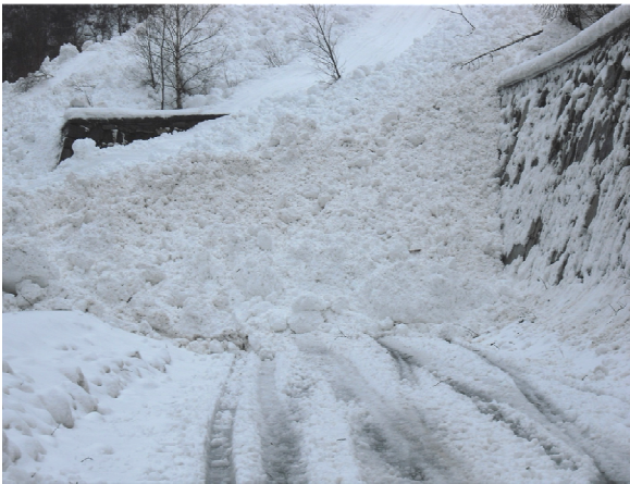
Figure 2: example of deposition area that blocks the tunnel entrance and obstructs the road for about 20 m.
