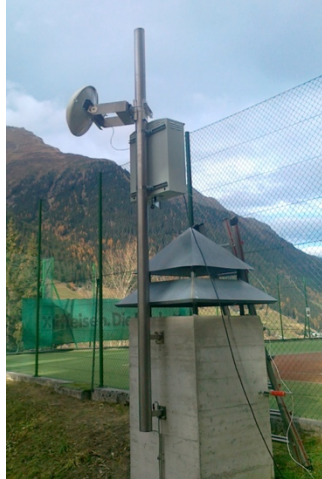
Figure 3: The radar device installed down in the valley facing the Großtal avalanche track in Ischgl, Austria.
