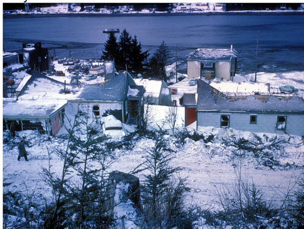
Fig. 4: View of Behrends Avenue with Gastineau Channel in the background after the 1962 avalanche – collapsed roofs because of overpressure and impacts of trees. The back-walls are not damaged (Alaska Mountain Safety Center).
