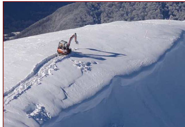
Figure.13: Excavators on Aibga ridge (Margreth, 2010)
