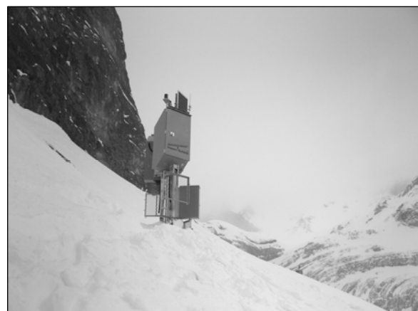
Figure 9: Avalanche Guard in waiting position.
