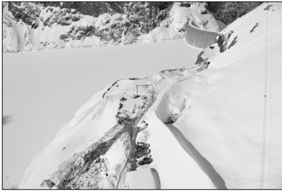
Figure 4. Dam against avalanches.
