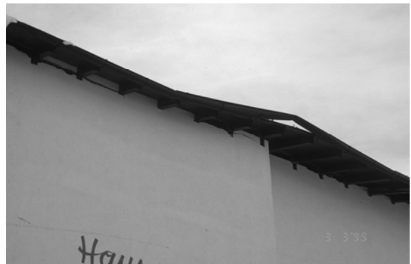
Figure 9. Damages on a roof caused by powder pressure
