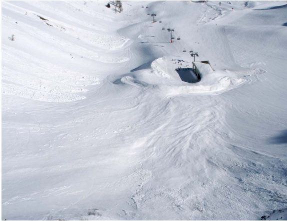
Figure 2: Top Station of the Chairlift 'Vaduzer Täli' on April 7, 2009. The Station is protected by a 3.5 m height curved earth dam, and the structure itself is designed to a maximum impact load of 86 kN/m 2 .
