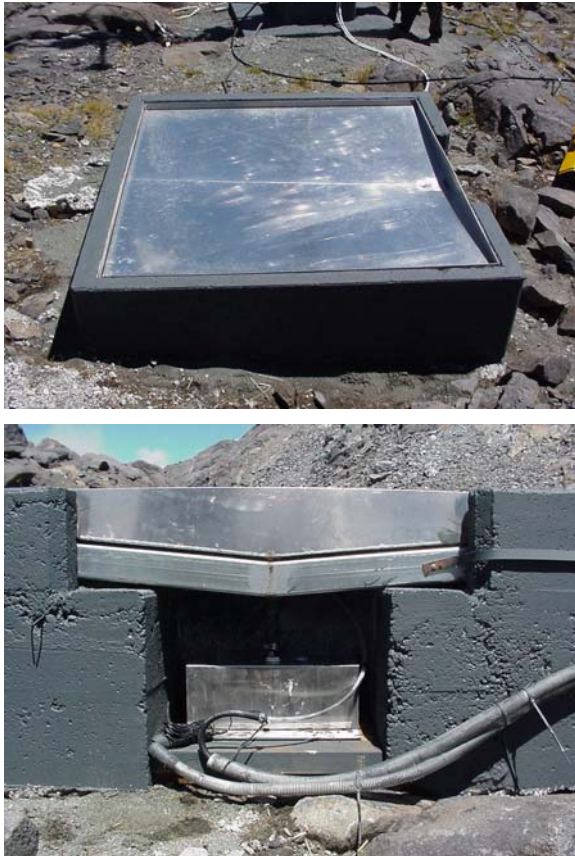
Figure 3: Summer pictures of the lysimeter at Belle (1600m). Upper picture shows the catchment tray. Lower picture shows the housing for the tipping bucket gauge. During winter the lysimeter is typically covered by 3-4m of snow.
