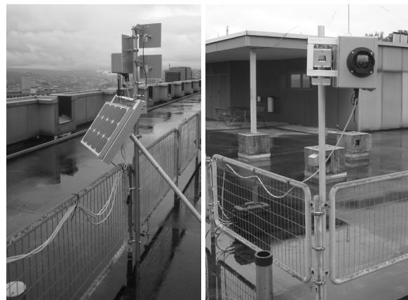
Figure 5. Rooftop testbed with base station, solar power system and long-range WLAN link (left). Camera is mounted in on a separate pole (right).
