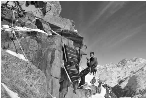
Figure 3. PermaSense base station including a solar power system and a Linux mini-computer located at 3500 m a.s.l. on the Hörnliridge, Matterhorn, Switzerland.
