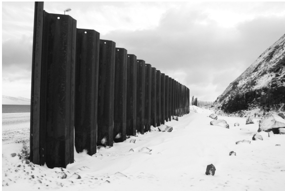
Figure 2. Steel sheet piles at Óshlíð in West fjords, Iceland. The wall is approx. 3 m high and is built to stop small avalanches and rocks before entering the road. Photo: Árni Jónsson 10/2005.
