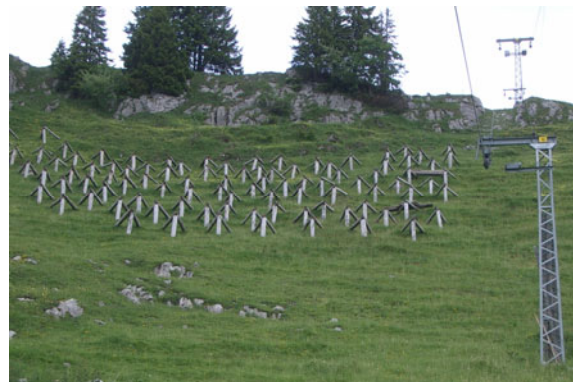
Figure 10: Tripod structures for the protection of the repaired mast 10 of the Bärenfall ski lift (case study 1).
