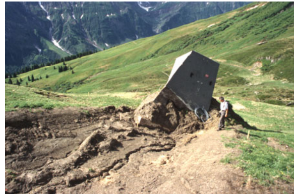
Figure 4: Destroyed foundation of mast 7 of the chairlift Pleus. The shallow foundation was displaced over more than 8 m (case study 2).
