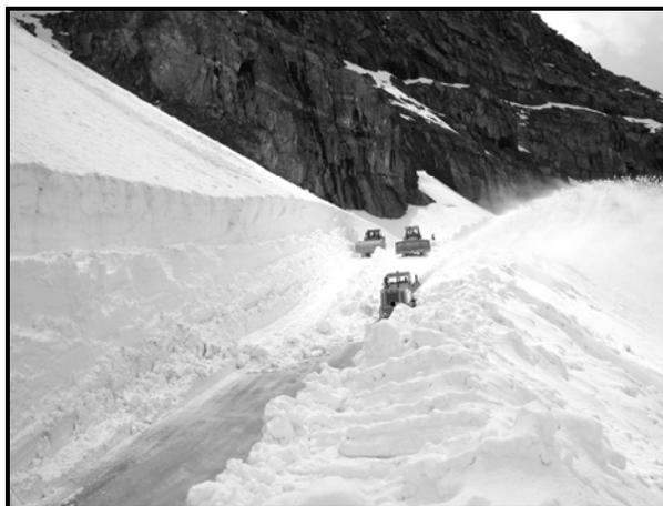
Figure 1: Dozers and rotary snow blower removing deep snow from Rimrock.
