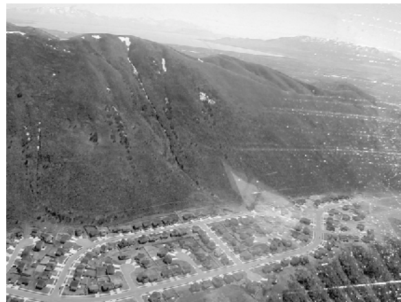
Fig. 6 This subdivision in was built below 40° slopes without consideration to avalanche hazard (prior to ordinance).
