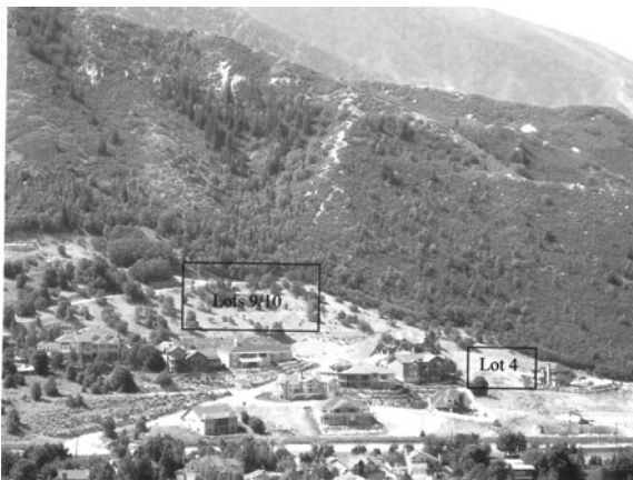
Fig 4 A typical area requiring a site-specific avalanche study - bottom of Little Cottonwood Canyon.
