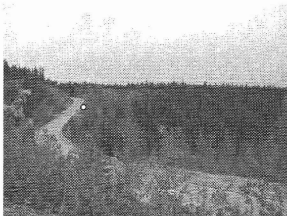
Figure 4. RWIS Station monitors hazard prone to gully due to its orientation, the road alignment, and potential for increased humidity from a creek at its base.
