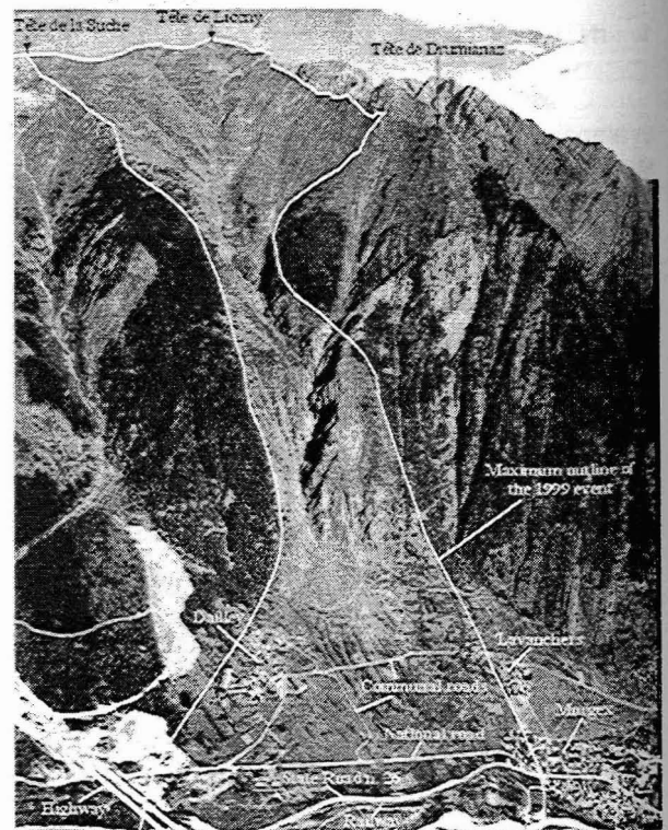
Figure 3: Aerial view of the Lavanchers site
