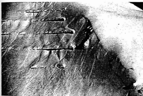
Fig. 11 Avalanche supporting structures at Chüenihorn above St. Antönien/GR, photographed on February 25 th , 1999. The photo shows clearly the effectiveness but also the limits of supporting structures with several loose snow avalanches on the surface of the snow pack (Foto SLF).
