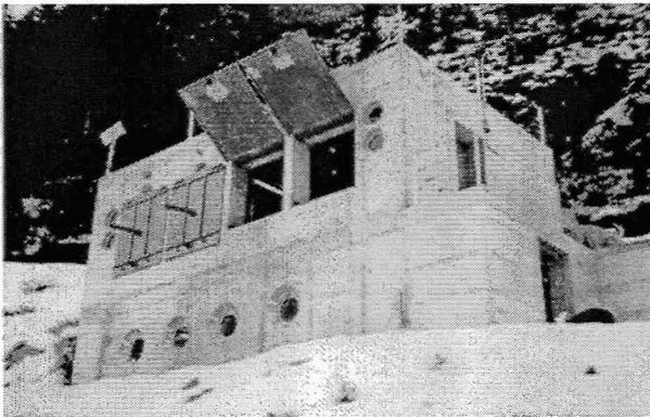
Figure 9 Shelter construction with observation portholes at ground level and the openings for the Doppler radars on the first level. The openings can fast and easily be closed to protect the radar equipment in case a powder-snow avalanche would hit the shelter
