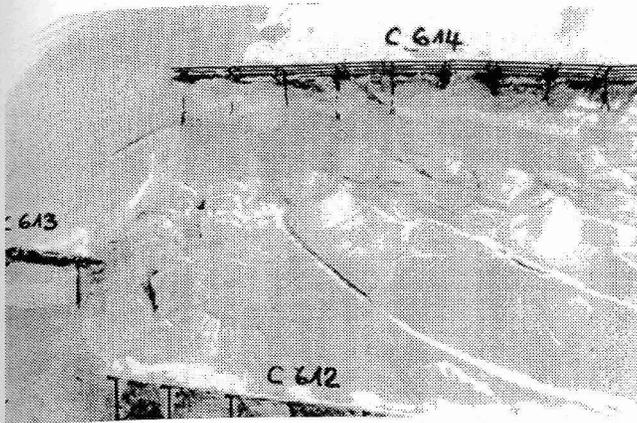
Fig.5: Hard slab stopped by steel bridges, Val Giandains-Pontresina
