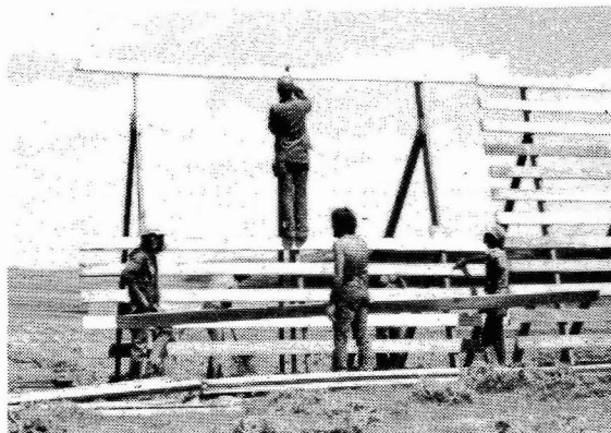
Figure 5. Truss-type fences are less expensive than post-supported fences.
