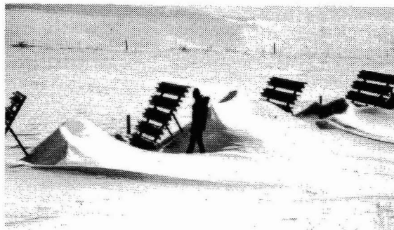
Figure 6. Leaving gaps in snow fences greatly reduces their storage efficiency.
