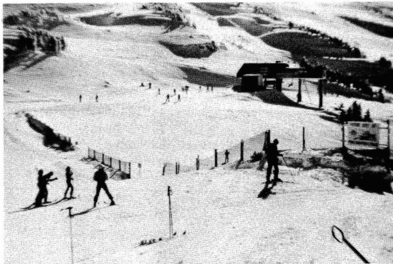
Figure 6 The snowfence provided a source of snow much nearer the problem area, allowing the lift to be used 2-3 weeks earlier and greatly improving snowcover around the landing throughout the 1987-88 winter.
