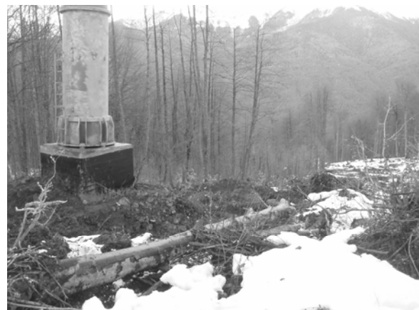
Figure 8: A chairlift tower adjacent to the Fin Path (D5) avalanche trimline.
