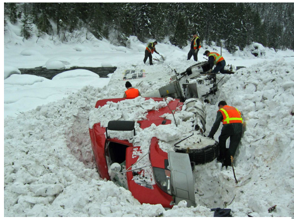
Fig. 5. Crews excavating the truck for removal from the Lochsa River.
