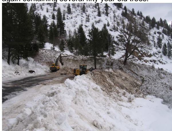
Fig. 7. This pile was 22' deep on the roadway. Rocks and trees in the debris made clean up difficult. This slide occurred during the second avalanche cycle, 2008. February 14, 2008
