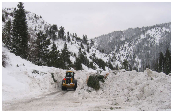
Fig. 6. Heavy equipment removing avalanche debris. February 7, 2008
