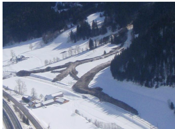
Figure 9: The railway track was submerged on a length of more than 500 m
