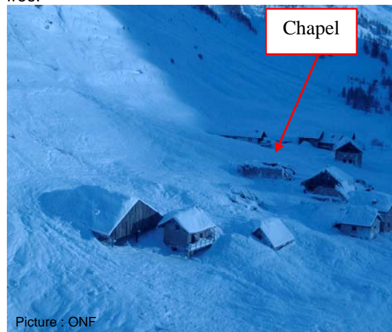
Figure 2: The chapel destroyed and houses damaged by an unknown avalanche in human memory.
