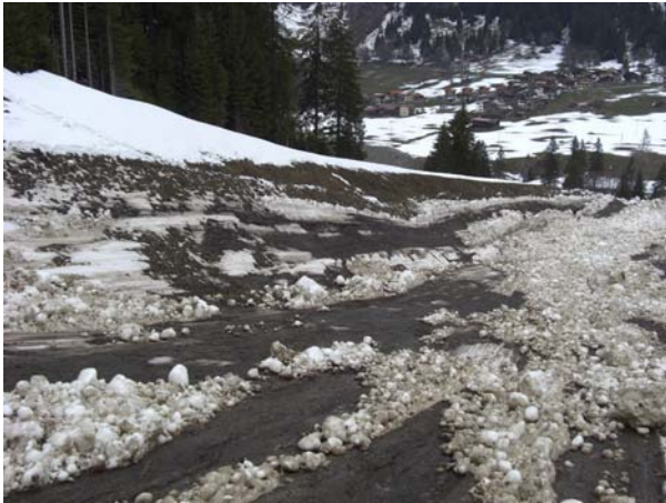
Figure 4. Avalanche run-up along the dam side facing the avalanche. Beside the dam location, the ground was the sliding surface of the avalanche.
