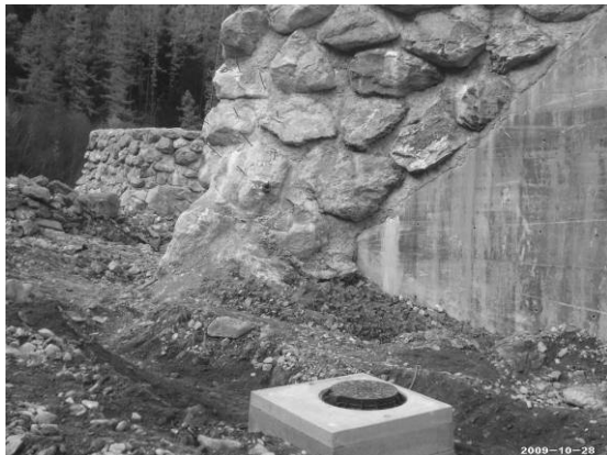
Figure 11 : Protective chamber for data logger at the foot of the breaking mounds
