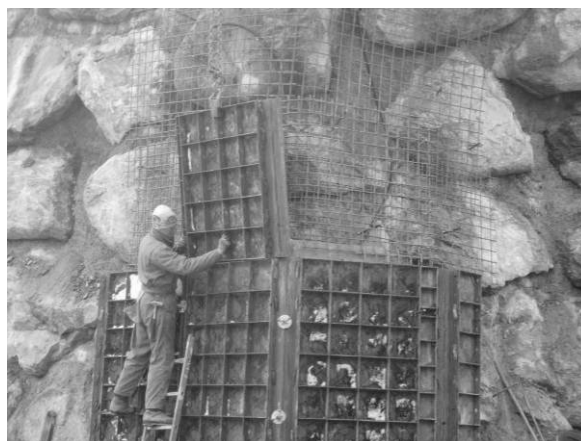
Figure 9: Reinforced concrete shear wall's building specially designed for supporting sensors and for withstanding flowing avalanche
