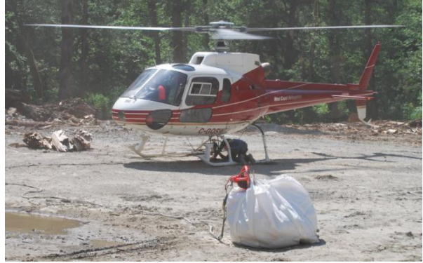
Fig. 11. 16 unprimed 25 kg ANFO bags ready for sling loading into the bomb crater.
