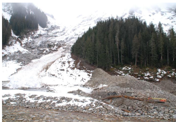
Fig. 8. Nearly completed deflection berm shown at right, Size 3 deposit shown in path at left for scale.
