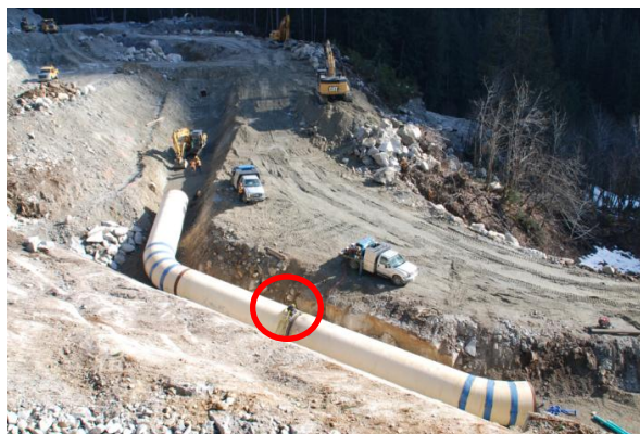
Fig. 12. Installing penstock along the Montrose Intake access road. Note welder on pipe in centre of photo (red circle), directly in an avalanche path.
