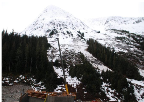
Fig. 13. Glide slabs located directly upslope of Montrose Intake worksite in Path MS-5.
