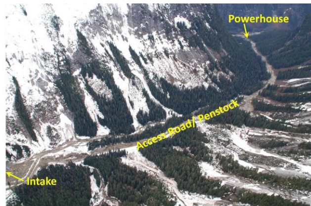
Fig. 3. Looking west down the Montrose Creek Valley towards Filer Creek and Powerhouse. Intake site is off left-hand side of photo.
