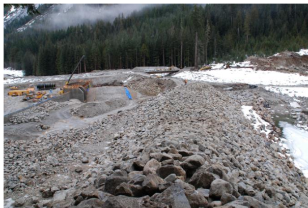
Fig. 7. Deflection berm at Montrose Intake. Photo taken looking north down the length of the berm, intake shown at left near the crane.
