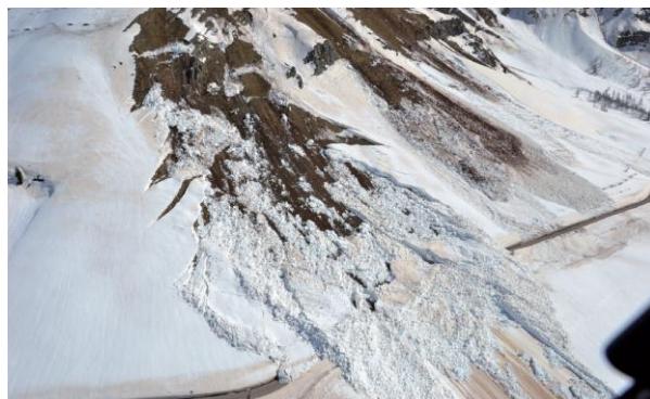
Fig. 18: national road n°. 50 at Passo Rolle interrupted the 16 th Mar. 2014 by several large full-depth and gliding avalanches - [courtesy Trento Province, 2014].
