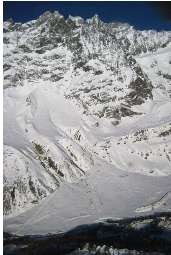
Figure 7. An image footage of n. 05_011 “Avouil (Hotel Carrel) - Becca de Guin SE” avalanche basin. On the right, the southern part of avalanche dam built to protect Breuil-Cervinia (photo: RAVA, 2013).
