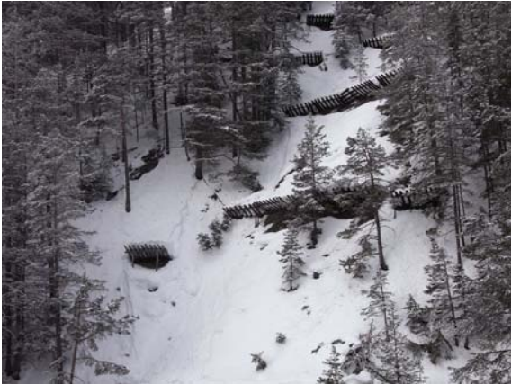
Figure 6: Forest avalanche starting zone located directly next to defense structures (photo: P. Caviezel).
