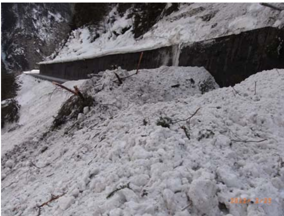
Figure 7: Road buried by an avalanche released from forest (photo: P. Caviezel).
