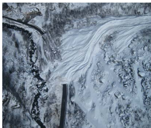
Figure 1. Regional route n. 44 (Aosta valley, Italy) (photo courtesy of UNV Aosta Valley).
