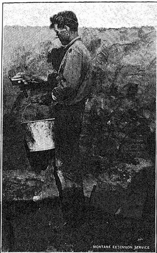
Putting on the whitewash coat of clear cement.
