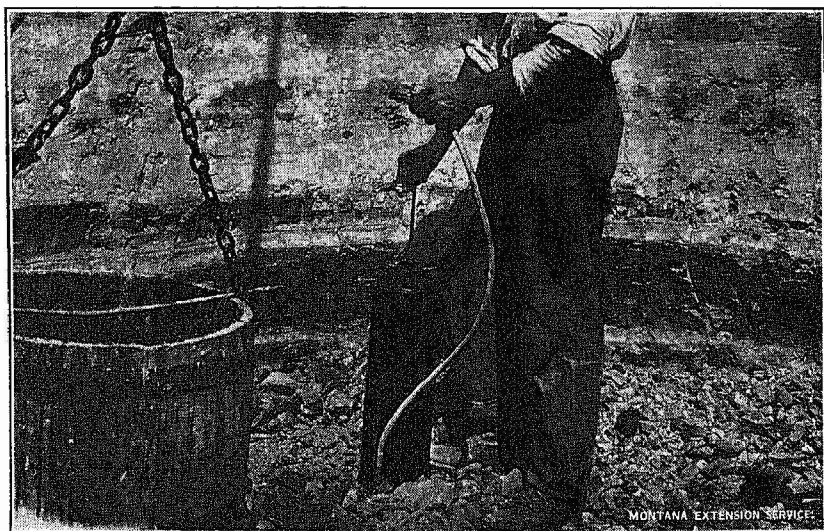
Moistening the walls before plastering.
